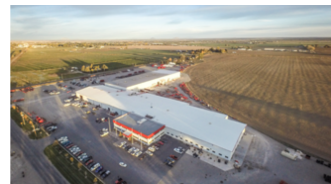
Spudnik Equipment Company LLC, Blackfoot, Idaho Headquarters and production site in North America.
